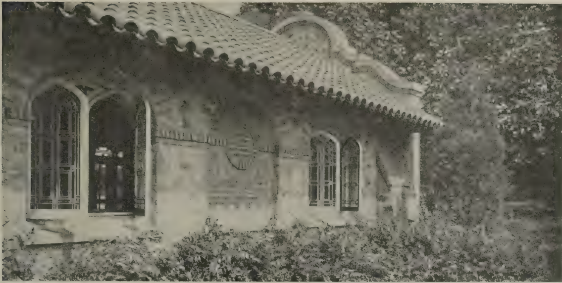
Fig. 10. Detail of a House at St. Davids, Pa. D. Knickerbacker Boyd, Architect
